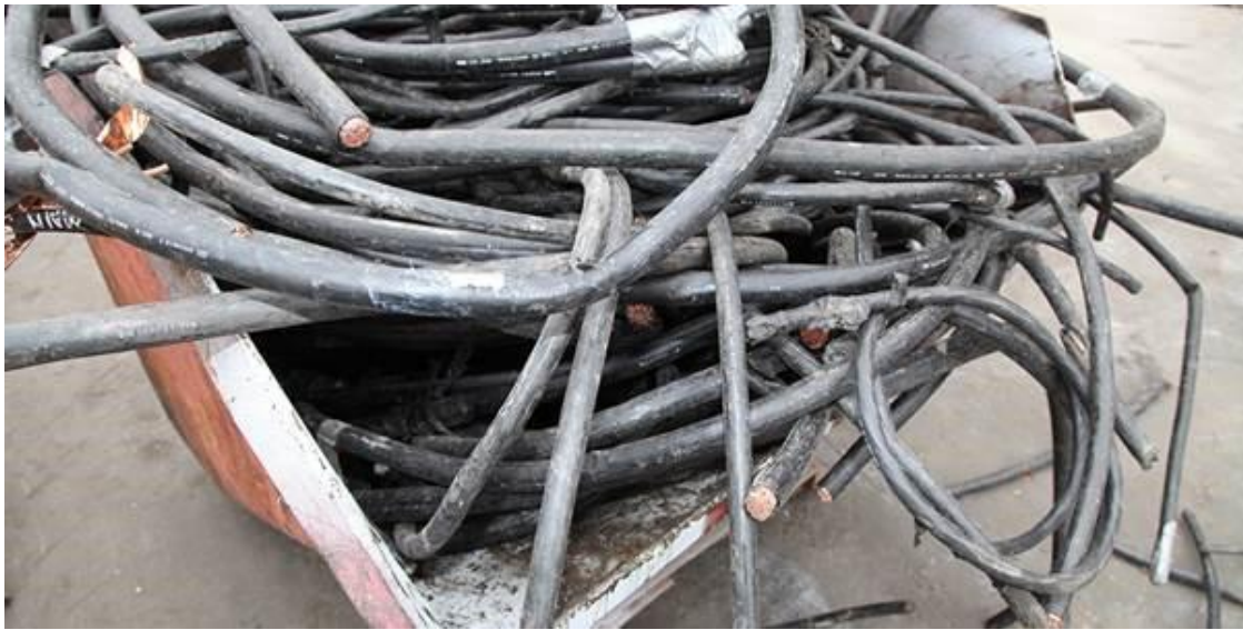
High Voltage Copper Cable is considered to contain 50% Copper.
